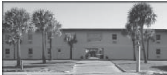
above : main entrance to renovated dormitory building
